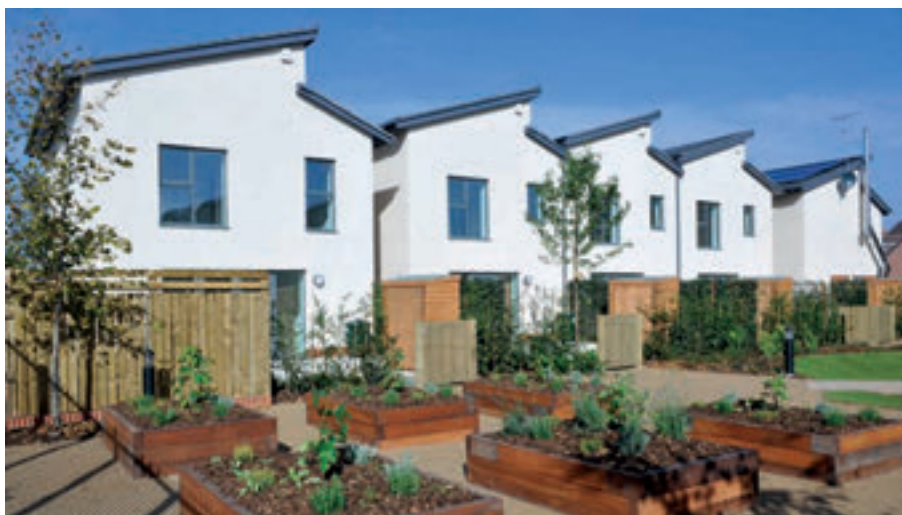
SSE's Greenwatt Way, a 'true' zero carbon home development built by Keepmoat
